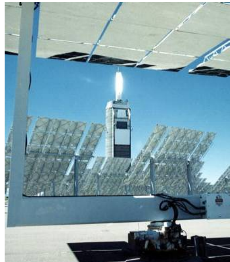
National Solar Thermal Test Facility
